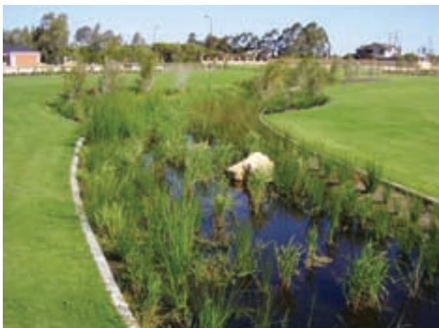
Photo 10: Inflow water flows through vegetated swale planted with sedges to remove nutrients from the water. There is also a concrete barrier separating the grass from the sedges restricting growth of both species and assisting in maintenance. However routine harvesting will still be required to control the growth of the sedges.
