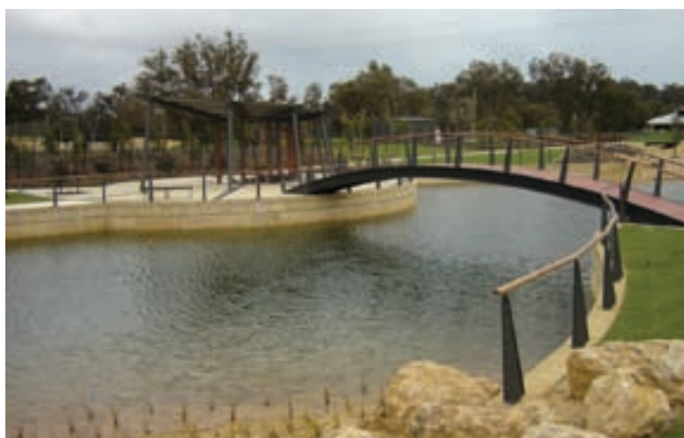
Photo 2: Shows hard vertical edges as well as barriers for public safety.
