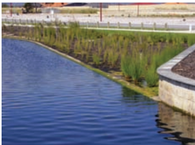
Photo 7: Sedge growth restricted to small pocket by concrete retaining wall
